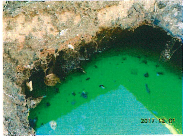
Elevated liquid level in tank during load test (baffle fallen away)
