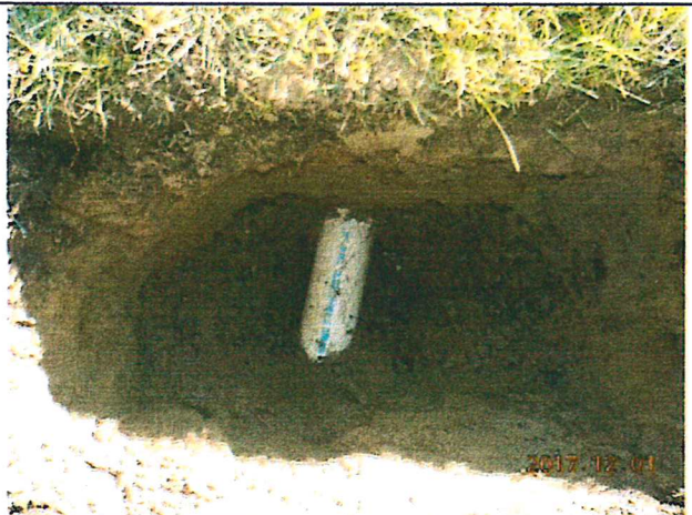
Distribution lateral line inside absorption trench (dry)
