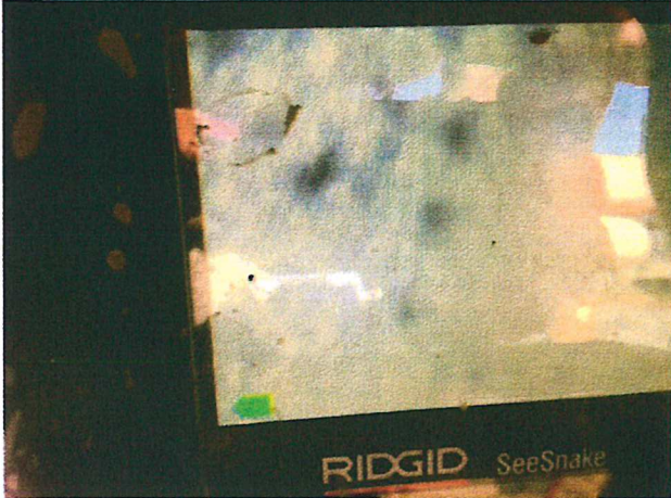
Outlet pipe between tank and leaching field (header) full of effluent
