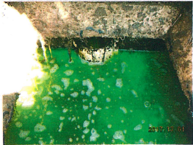
Plastic shield inlet baffle (green tracer dye in tank)
