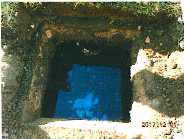
Outlet access and plastic shield baffle
