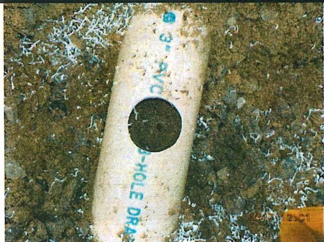
Hole in pipe showing line full of sediment
