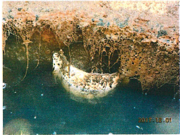
Outlet baffle falling away from tank wall
