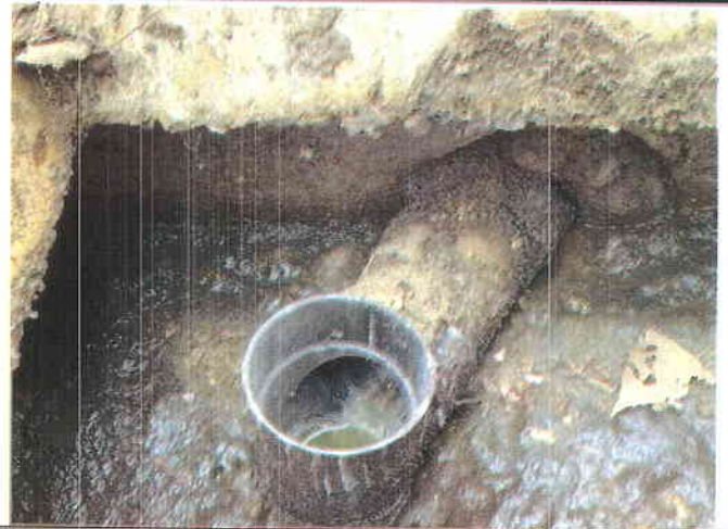
14. Septic tank outlet – baffle detail
