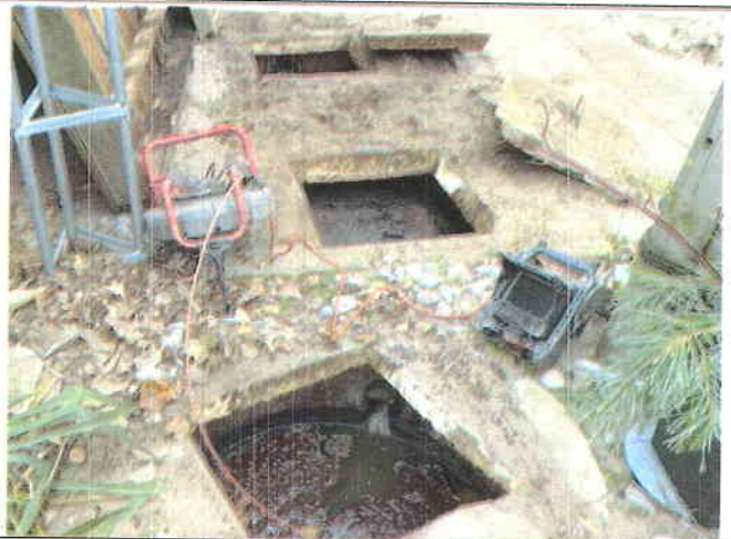
6. Septic tank and pump chamber configuration
