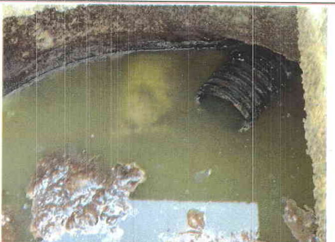
18. Pump chamber – corrugated 'Big-O'
