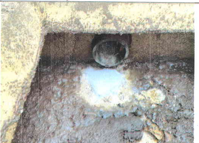
12. Septic tank inlet – detail
