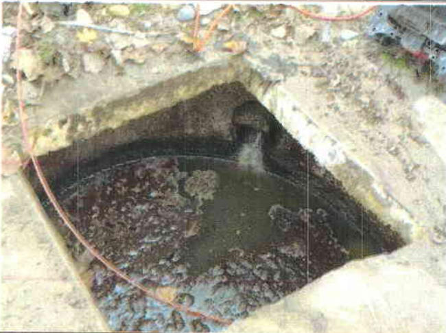
15. Pump chamber – with sewer line inspection camera
