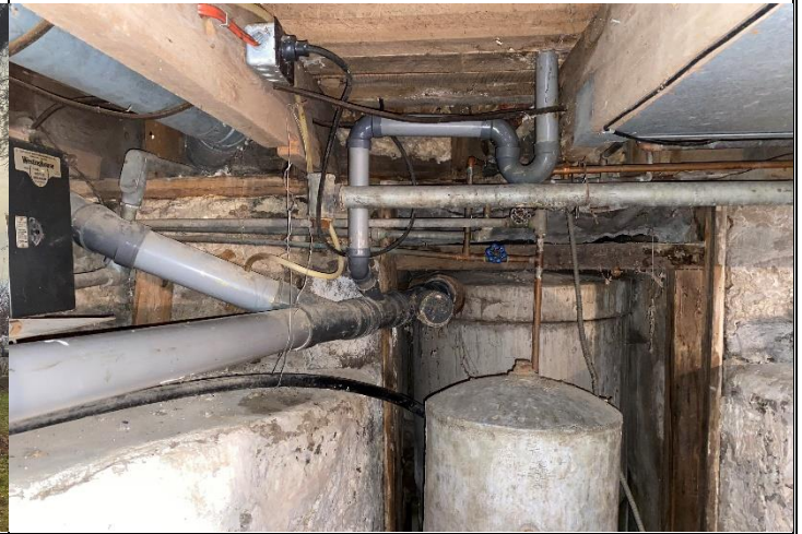
2. Sewer line inside home – well casing also visible
