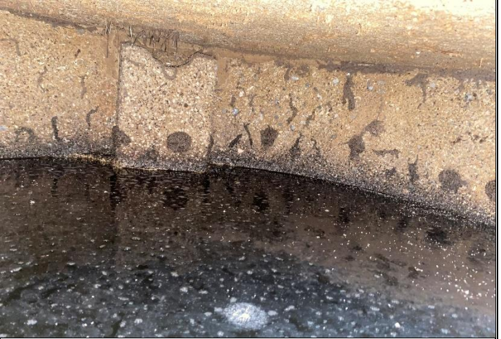
8. Interior of septic tank – inlet baffle visible
