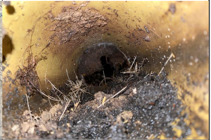
14. Interior of leaching field piping – moderate solids accumulations and root intrusion
