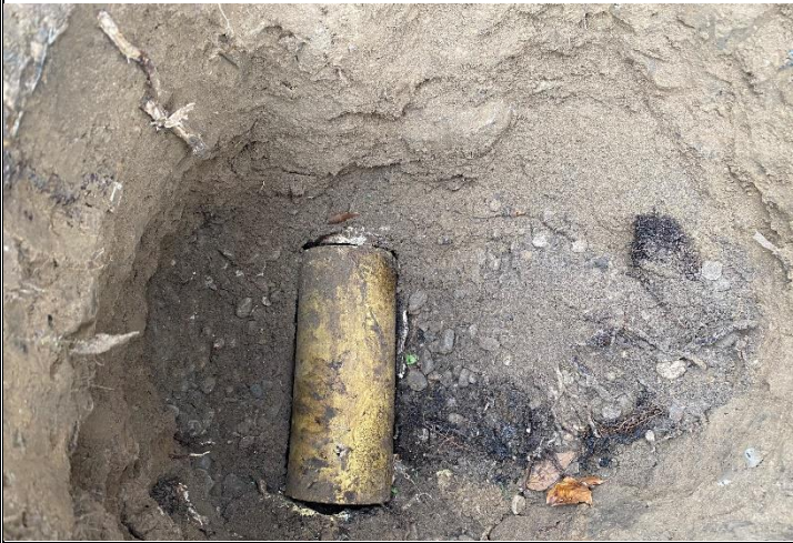
13. Excavation made to access leaching field – clay tile visible
