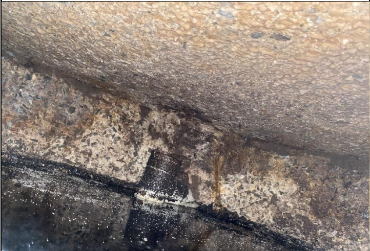
9. Interior of septic tank – outlet baffle visible
