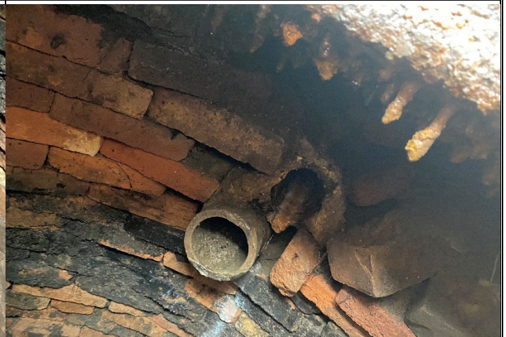
6. Sewer line entering the pit
