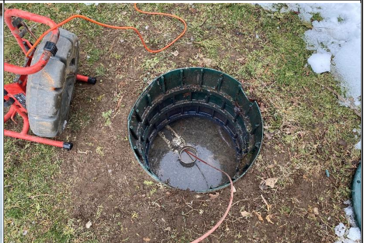
6. Camera inspection of discharge line
