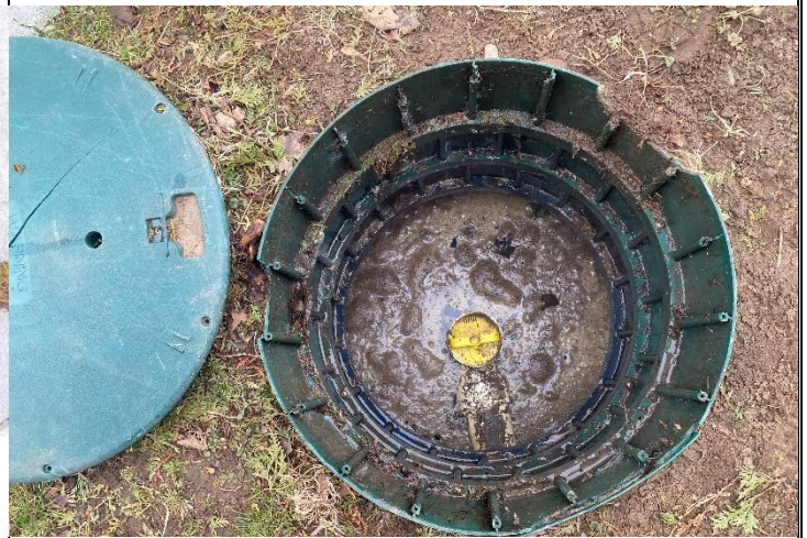
4. Septic tank outlet – clean effluent filter every 6 months
