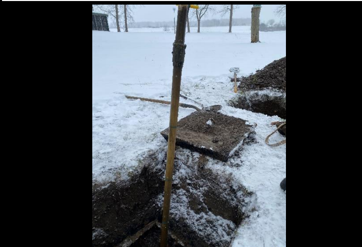
5. Septic tank solids measurement – pump out required.
