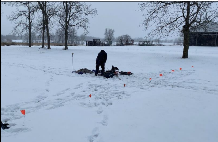
9. Septic tank and portion of leaching field with distribution laterals flagged.
