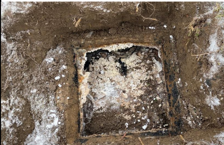
3. Septic tank outlet compartment – outlet baffle deficient.
