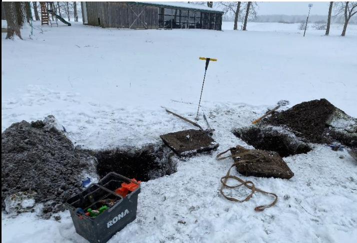
1. Septic tank location – lids buried ~1.5 ft. below grade.
