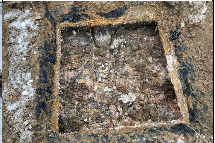
2. Septic tank inlet compartment – inlet baffle functional.
