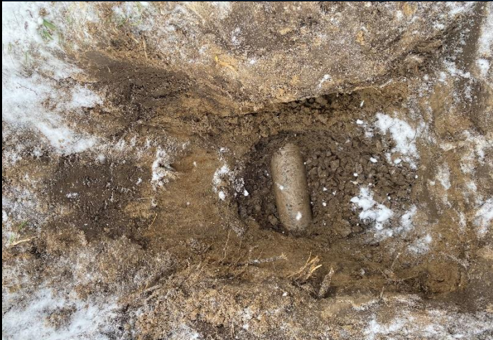
7. Leaching field excavation test pit revealed satisfactory soil conditions – distribution lateral visible.
