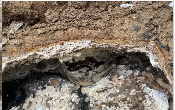
4. Outlet baffle detaching from septic tank wall & allowing solids to pass through into discharge pipe.
