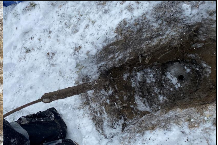
8. Camera covered in sludge upon entry of distribution lateral – leaching bed flush highly recommended.
