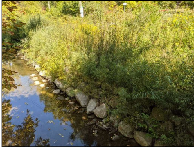
Photo 4: Example of a vegetated buttress.
